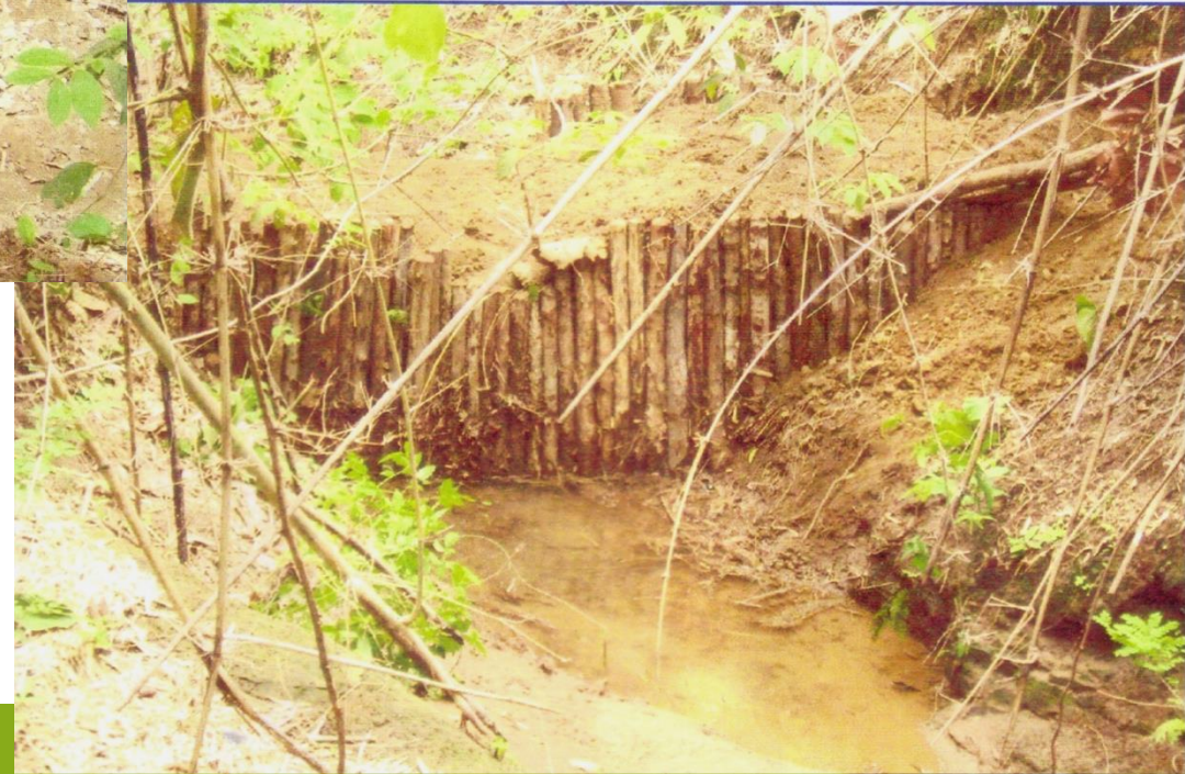
Check-dam (Pole & soil)
